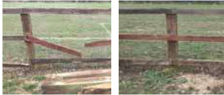
Part of fencing before Part of fence repaired
